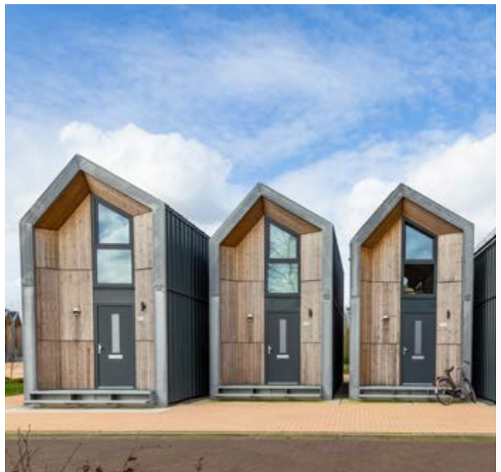
Eco friendly tiny houses in Nijkerk, Netherlands
